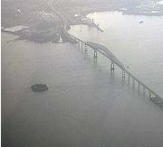
Fort Carroll, next to the Key Bridge in Baltimore, Maryland
