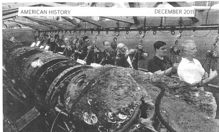
H.L. Hunley project staffers and volunteers rotate the sub using come-along winches.
